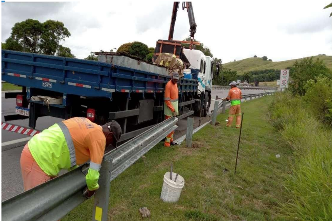
Figura 6.7 Via Lagos – Reparo Defensas – Km 17+500 Sul
